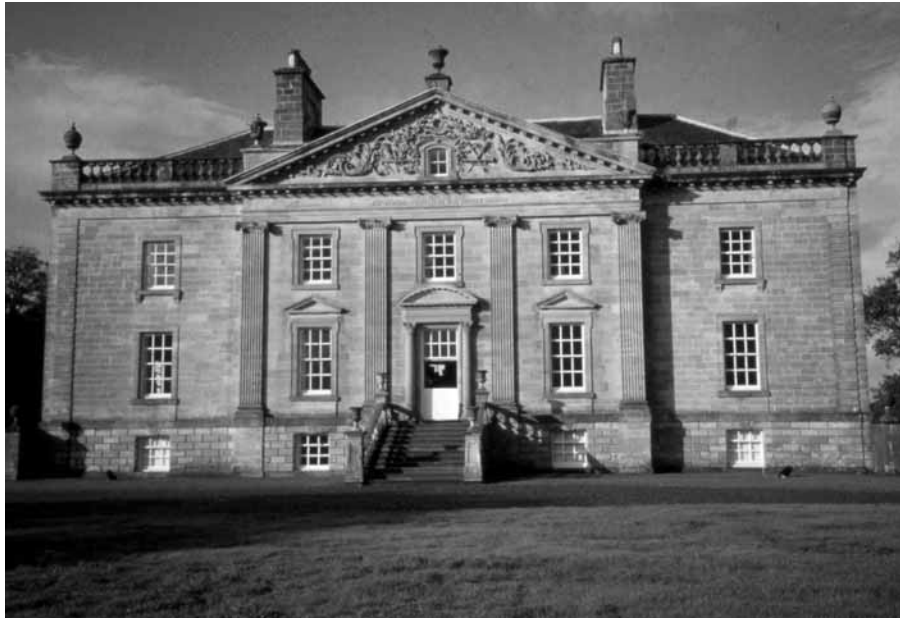
Auchinleck House today. It was built about 1760 by Alexander Boswell, Lord Auchinleck. This image is courtesy of the Landmark Trust, from whom it is available to rent as well as tour.
